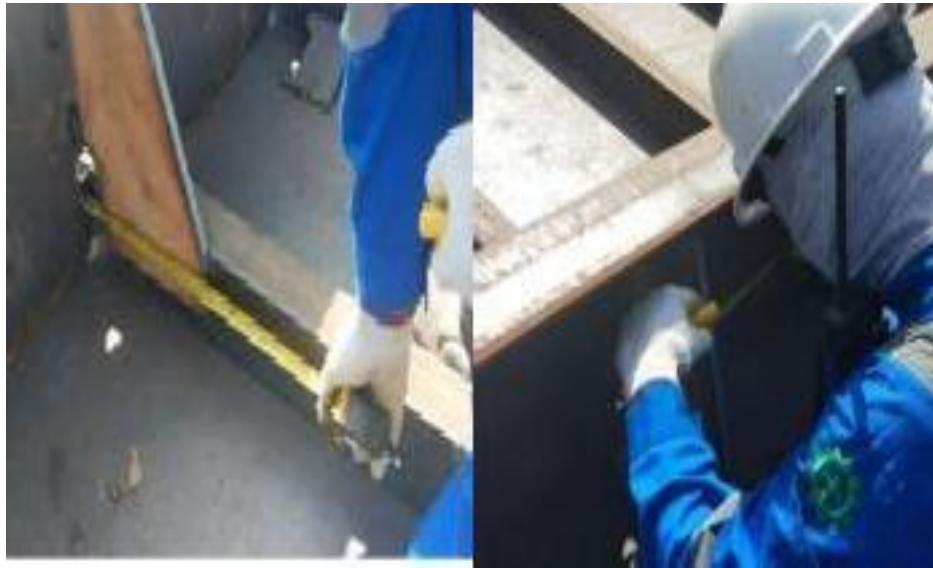
Gambar 2. 105 Fit Up Insect H-567
