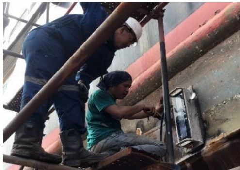
Gambar 2. 28 Proses vacuum test
