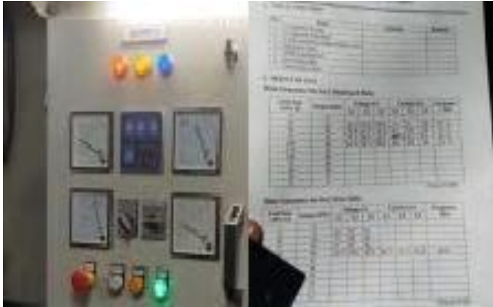
Gambar 2. 80 Load Test by BKI
