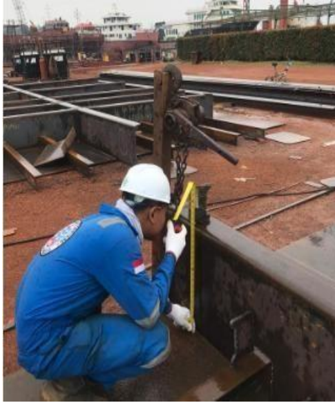
Gambar 2. 13 Hasil fit up check
