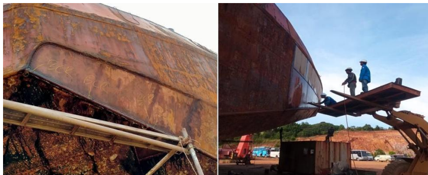
Gambar 2. 77 Air Test Void tank tongkang repair
