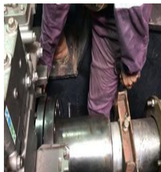
Gambar 3. 5 Proses Shaft Alignment
