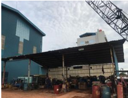
Gambar 1. 10 Workshop Mechanical & Electrical
