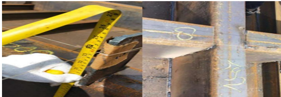
Gambar 2. 4 Hasil fit up check
