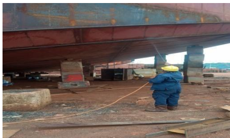
Gambar 2. 123 Air test tongkang repair
