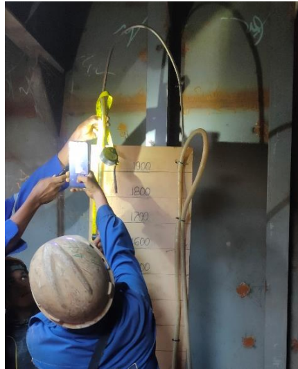
Gambar 3. 1 Air Pressure Test
