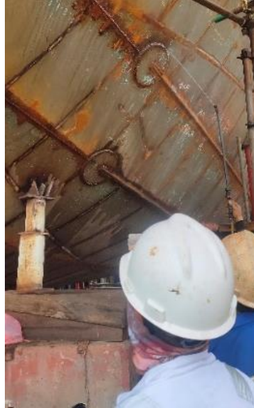
Gambar 2. 32 air pressure test
