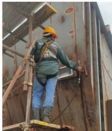
Gambar 2. 31 vaccum test
