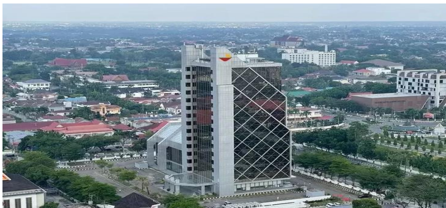
Figure 2.1 Dang Merdu Tower of Bank Riau Kepri Syariah Source: riau.harianhaluan.com
