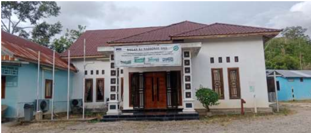
Figure 2.1 Site Office PT. Sorikmas Mining Malintang Source: PT. Sorikmas Mining 2022
