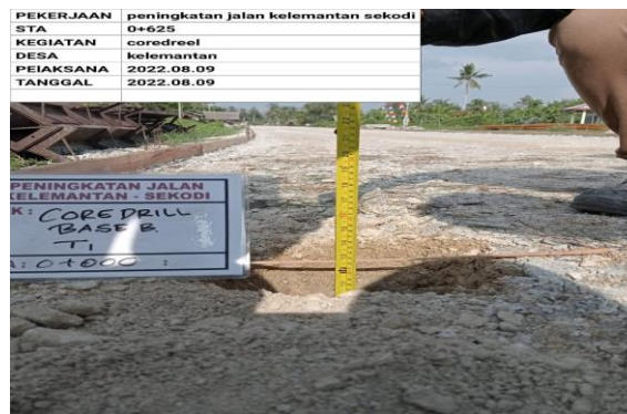
Gambar 3. 21 uji core drill
