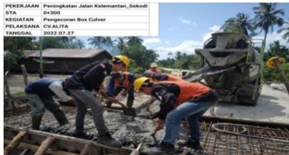
Gambar 3. 13 pengecoran box culvert
