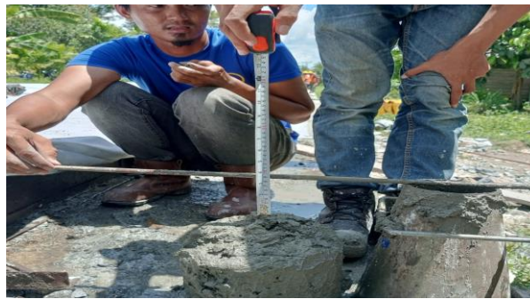
Gambar 3. 28 uji slump test
