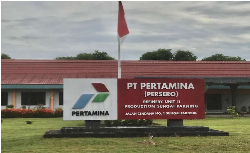
Figure 3.13 Workshop of PT Kilang Pertamina International Refinery Unit II Production Sungai Pakning
