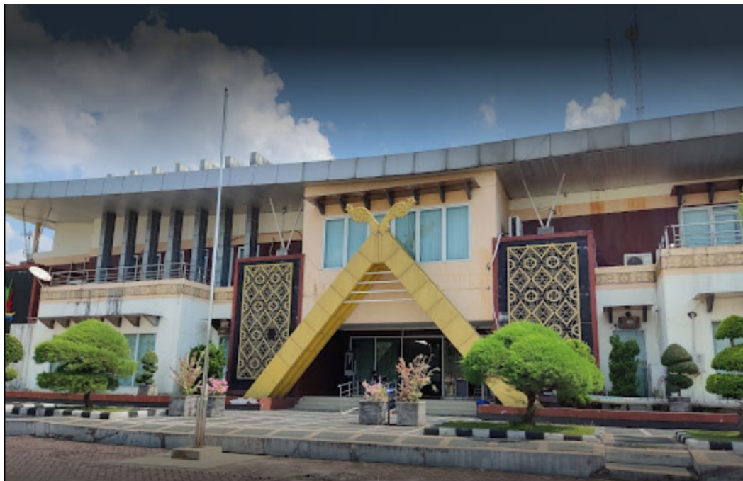
Figure 2.1 The Building of Tourism Office of Riau Province
