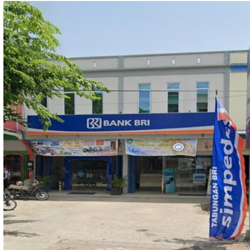
Figure 3.1. BRI Bengkalis Sub Branch Office
