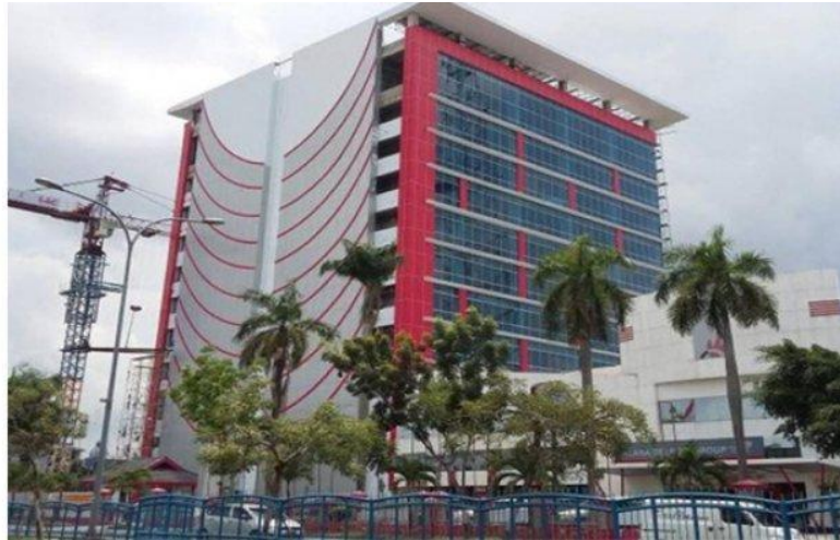
Figure 1.1 Graha Merah Putih Building of Pekanbaru Source: Telkom Website, 2023
