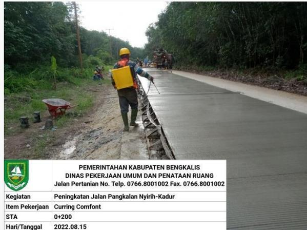
Gambar 3.17 Penyemprotan *Curing Compound*
