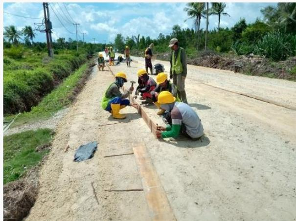
Gambar 4.6 Pemasangan Bekisting LC
