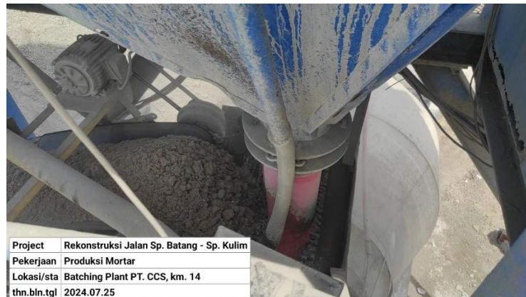
Gambar 3. 5 Pencampuran Material kedalam Truck Mixer di Batching Plant
