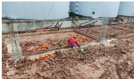
Gambar 3.19 Pemasangan Bekisting Bata *Ground Beam*
