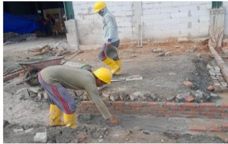
Gambar 3.18 Pemasangan *Lean Concrete Ground Beam*
