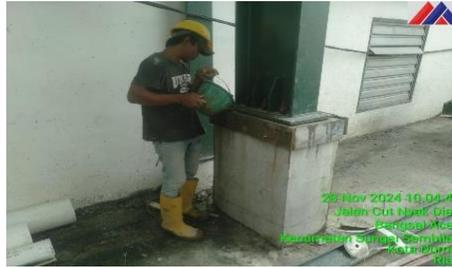
Gambar 3.46 Grouting Pedestal
