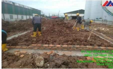
Gambar 3.22 Penimbunan Tanah Kembali *Slab* Beton
