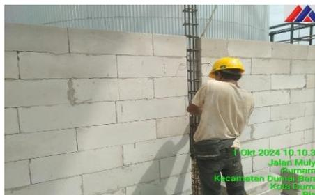
Gambar 3.48 Instal Round Bar dan Kolom Praktis Dinding Bata
