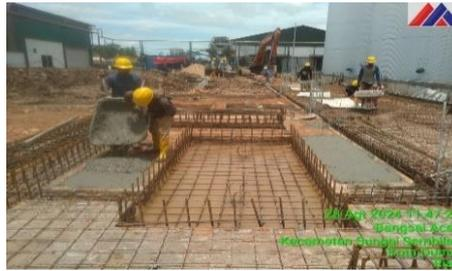
Gambar 3.25 Pemasangan *Lean Concrete* Slab Beton
