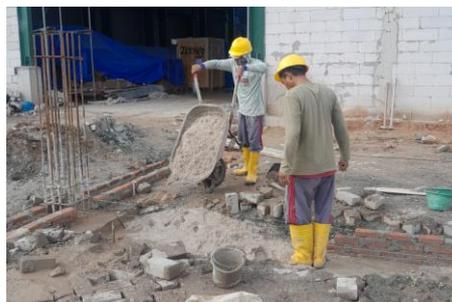
Gambar 3.17 Pemasangan Urugan Pasir *Ground Beam*
