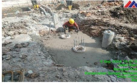
Gambar 3.37 Pemasangan Lean Concrete Dudukan Equipment
