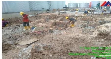
Gambar 3.38 Pemasangan Bekisting Dudukan Equipment
