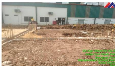
Gambar 3.24 Urugan Pasir *Slab* Beton
