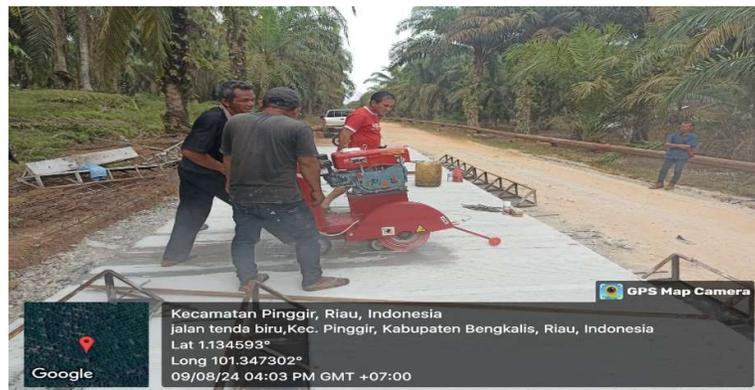
*Gambar 3 31. Pemotongan Beton (Cutting)*
