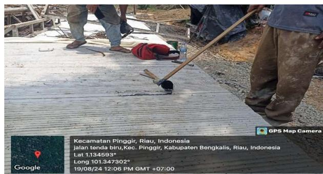
*Gambar 3 32. Penuangan Joint Sealant*
