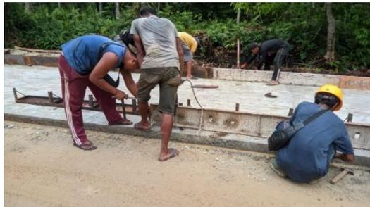
Gambar 3. 12 Pemasangan besi penahan mal rigid
