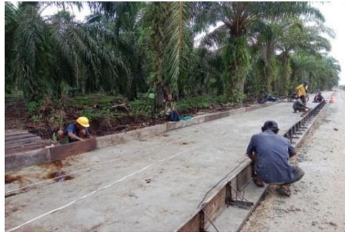
Gambar 3. 13 Pengikatan besi penahan bekisting rigid
