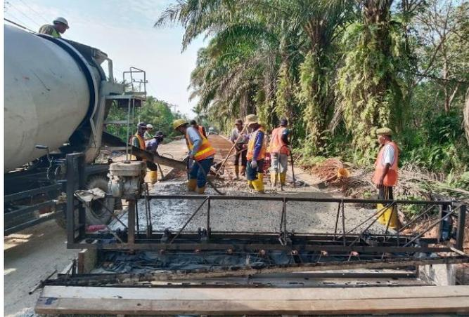
Gambar 2. 9 Truss Screeder Dynamic
