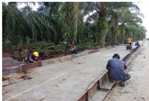
Gambar 3. 13 Pengikatan besi penahan bekisting rigid
