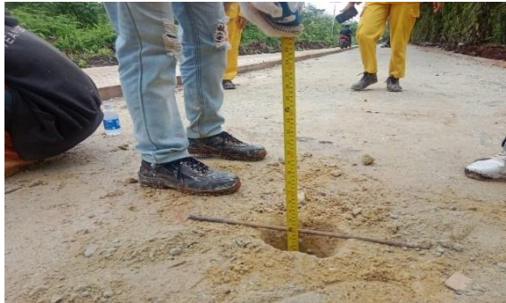
Gambar 3. 7 Penegcekan Ketebalan Base B
