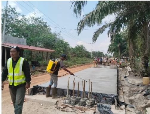
Gambar 3. 22 Pekerjaan Curing Compound
