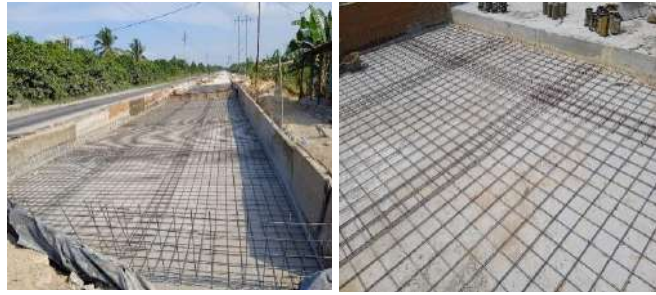
Gambar 3. 10 Penulangan Wiremesh
