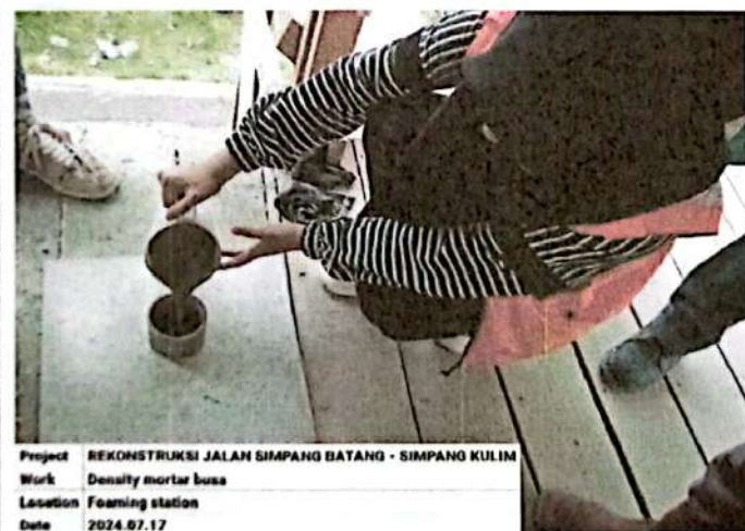
Project REKONSTRUKSI JALAN SIMPANG BATANG - SIMPANG KULIM Work Density mortar busa Location Foaming station Date 2024.07.17
