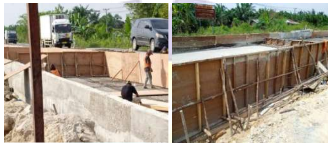
Gambar 3. 7 Bekisting badan jalan
