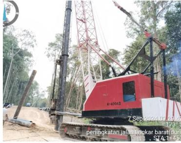
**Gambar 3. 6 Diesel Hammer**
