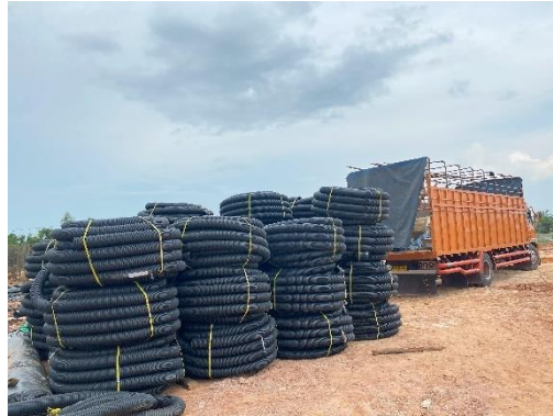
Gambar 3.67 Pegadaan Pipa HDPE Perforated Corrugated Dia 4 (Sumber: Dokumentasi Lapangan, 2024)
