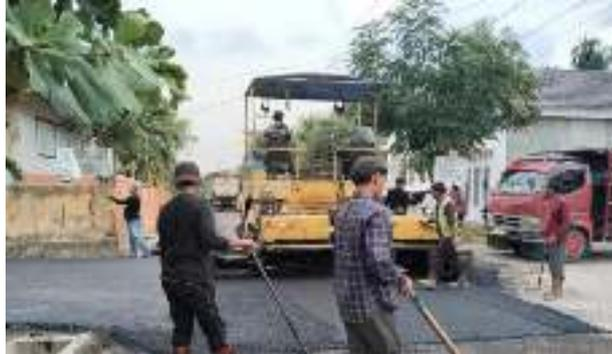
*gambar 3. 5 Asphalt Finisher*
