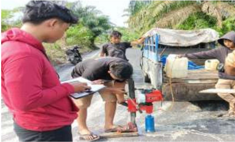
*gambar 4. 17 Core Drill*
