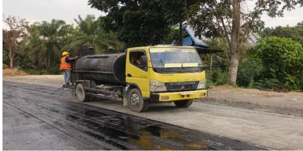
**Gambar 3. 6 Asphalt Sprayer Truck**
