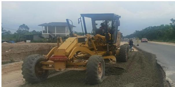
**Gambar 3. 3 Alat Berat Motor Grader**
