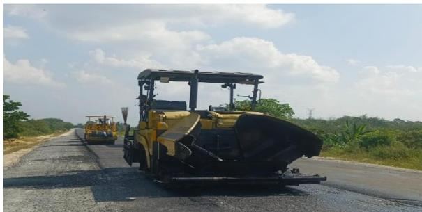
**Gambar 3. 7 Asphalt Finisher**
