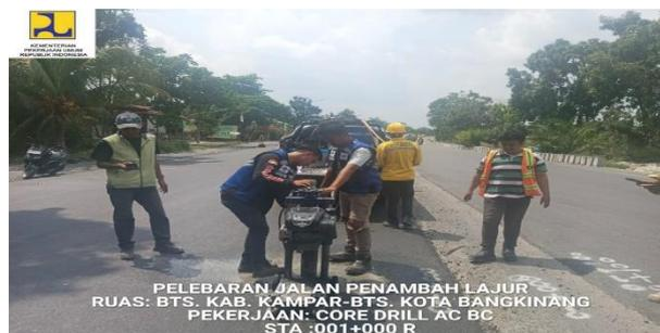
**Gambar 3. 25 Core Drill Aspal AC-BC**
