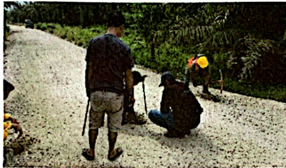
Gambar 4.5 Penge-Core-An Base A
