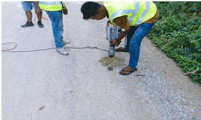
Gambar 3 22 pekerjaan core drill base A
