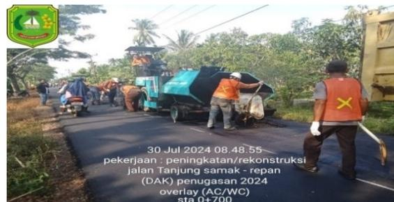
Gambar 3 9 Asphalt Finisher
