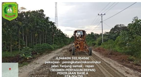
Gambar 3 3 Motor Grader
