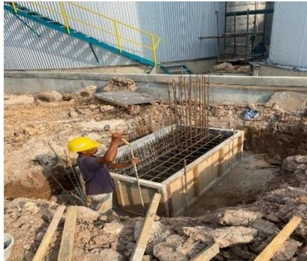
Gambar 3.38 Proses marking Top cor pondasi F1
