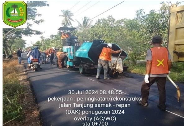
*Gambar 1. 12 Asphalt Finisher*
