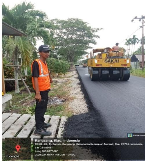
*Gambar 1. 14 Pneumatic Roller*
