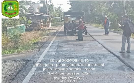
*Gambar 1. 11Asphalt Sprayer*
