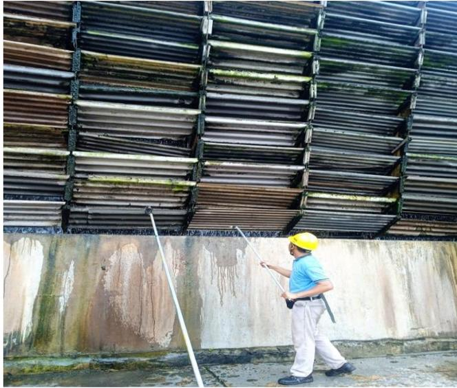
Gambar 2. 19 *Cleaning Louver Cooling Tower*
