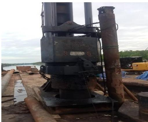
**Gambar 4. 14** Hammer Diesel
