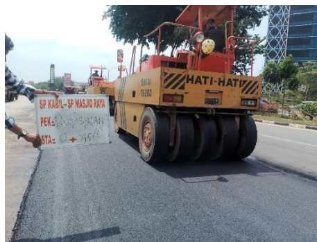
Gambar 3.24 Pneumatic Roller
