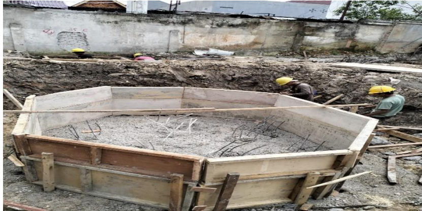
Gambar 3. 7 Proses perakitan bekisting
