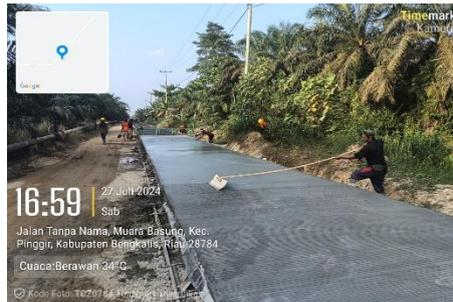
*Gambar 3. 19 Grooving beton
