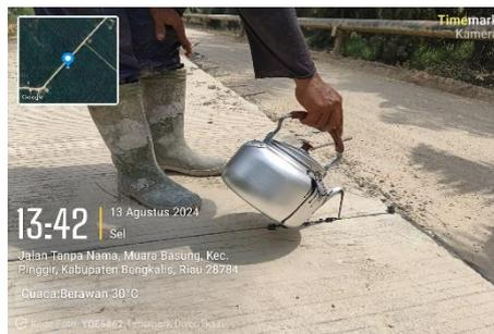
*Gambar 3. 21 Joint sealant
