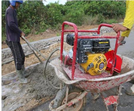
*Gambar 4. 3 Concrete Vibrator
