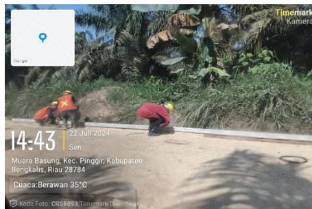
*Gambar 3. 11 Pemasangan Bekisting LC
