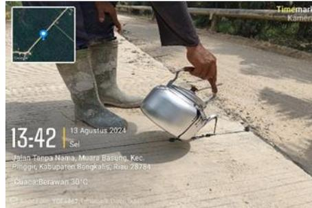
*Gambar 4. 29 Joint Sealant
