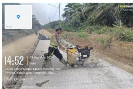
*Gambar 4. 28 Cutting Beton
