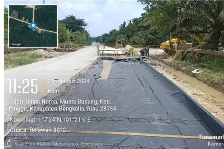
*Gambar 4. 13 Pemasangan Crack Inducer
