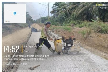
*Gambar 3. 20 Cutting beton
