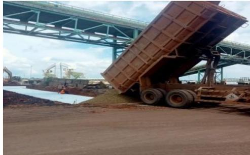
**Gambar 3. 12** Proses Penimbunan Material Quarry Waste
