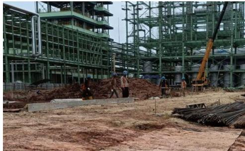
**Gambar 3. 14** Proses Pemasangan String line
