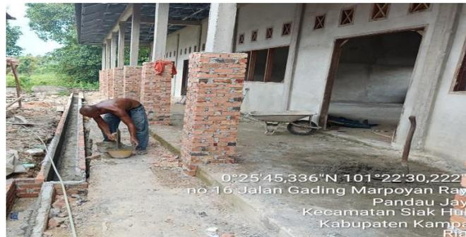
Gambar 3. 28 Plasteran Kolom Teras
