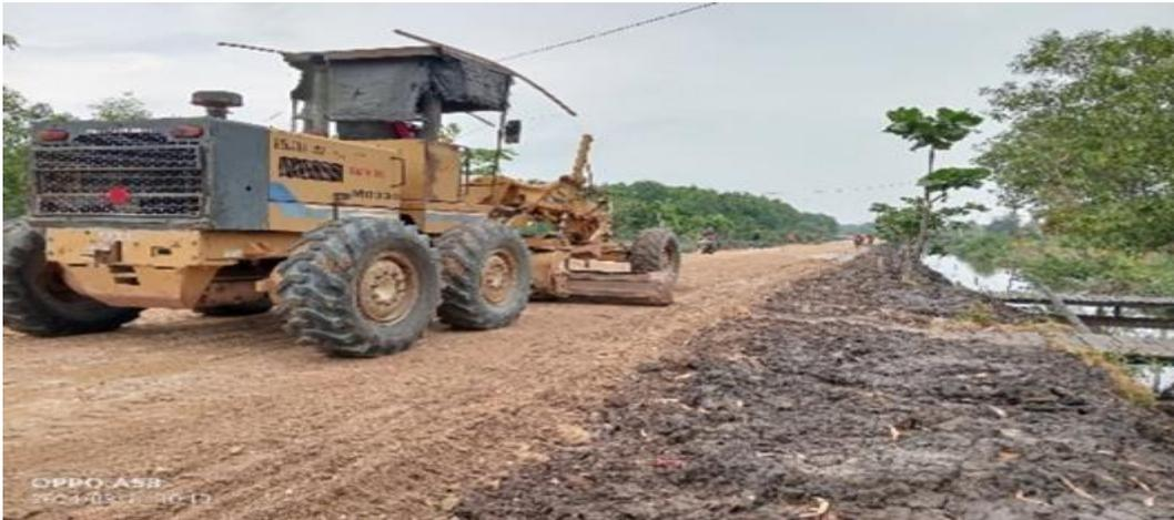
**Gambar 4. 4** Passing Motor Grader
