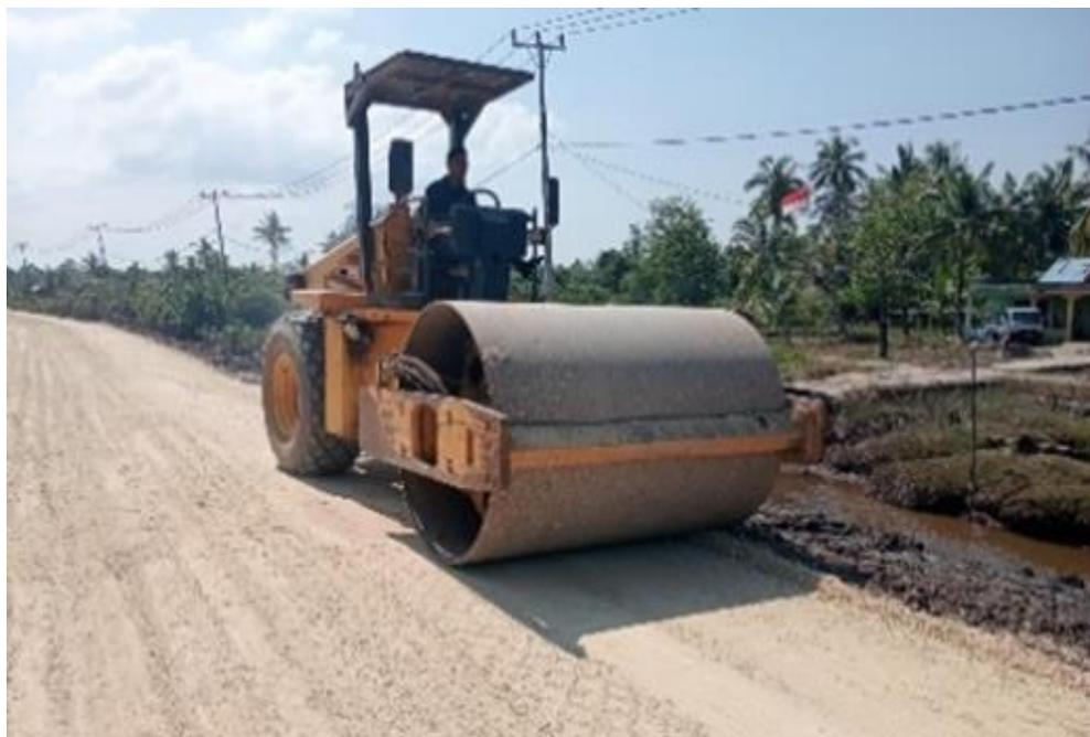
**Gambar 3. 3** Gambar Vibratory Roller
