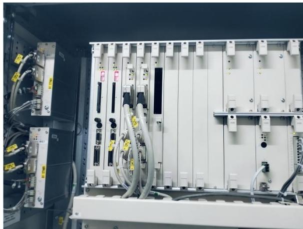
Gambar 3. 3 ABB Controller AC450
