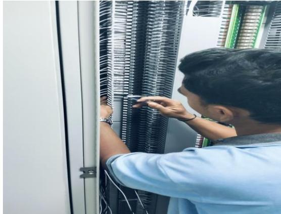
*Gambar 2. 3 connect cable to terminal block*
