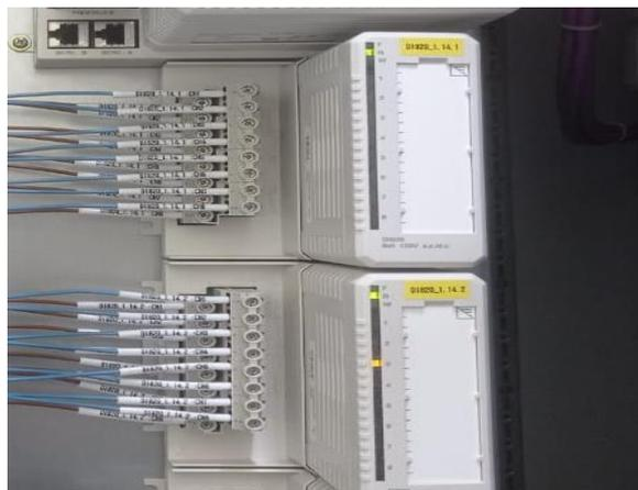
Gambar 3. 6 ABB Controller D180
