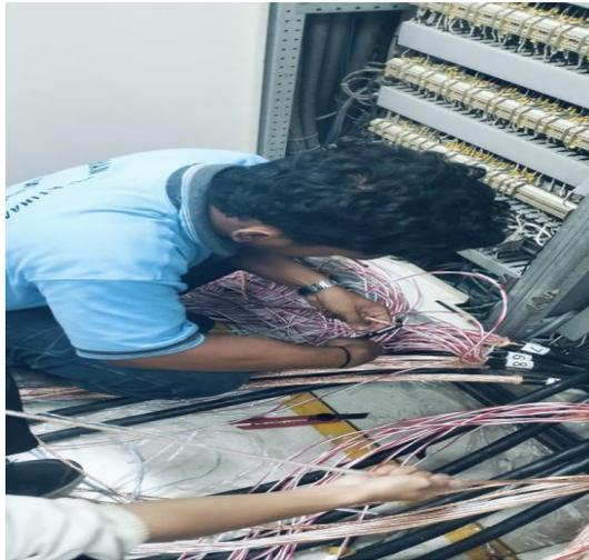
*Gambar 2. 2 Stripping of channel cable*
