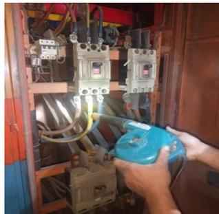
**Gambar 3.15 Cleaning panel engine room**
