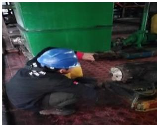
**Gambar 3.38 Cleaning elektro motor 3 phasa**
