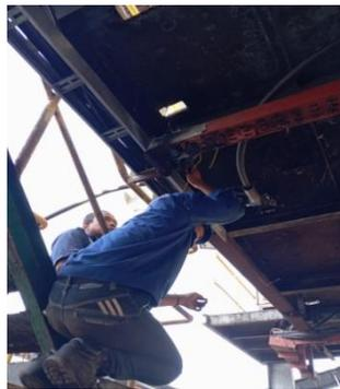
**Gambar 3. 95 Pemasangan kabel *connect* panel autotrafo**
