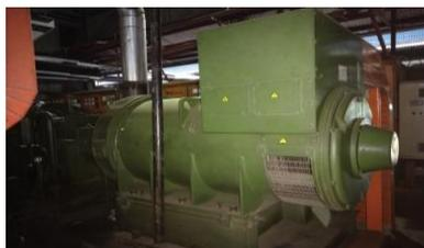
**Gambar 3.1 Generator PLTU boiler**
