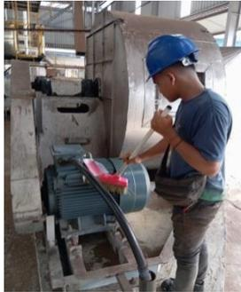
**Gambar 3.113 Cleaning elektro motor**
