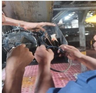
**Gambar 3.90 Penggantian elektro motor *coveyor buttom threshing***
