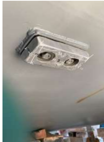
CONTOH GAMBAR CATHODIC PROTECTION
