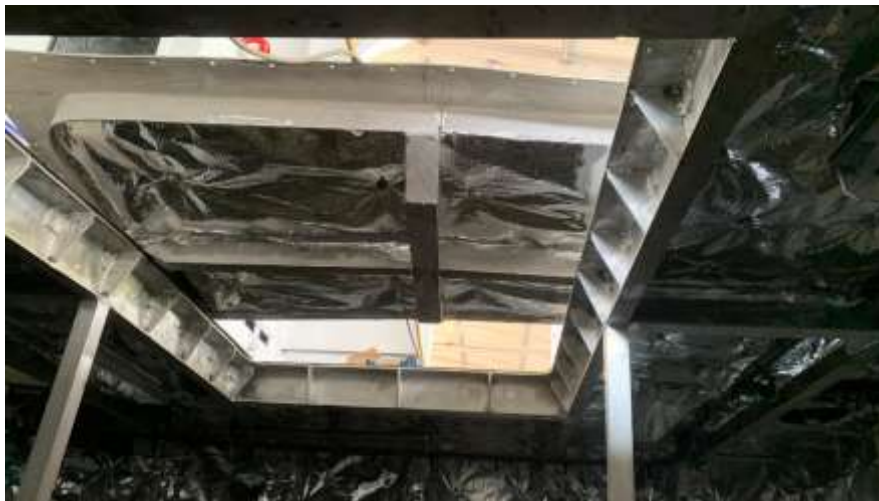
RUANGGAN ENGINE ROOM
