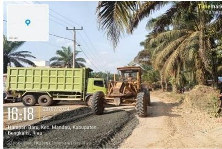
Gambar 3. 3 Motor Grader
