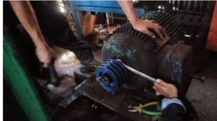
**Gambar 3. 56 Ganti pulli motor press**
