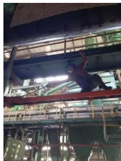
**Gambar 3. 9 Pengecatan panel treay cable karnel**
