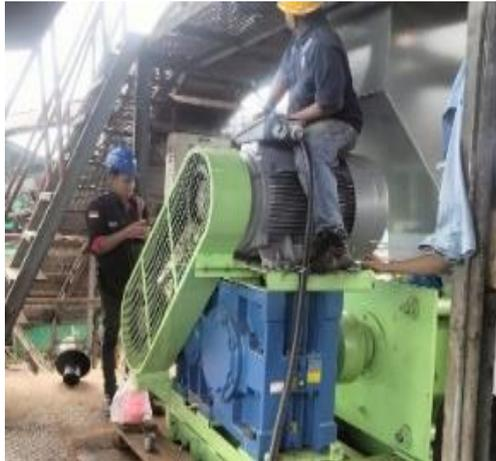
**Gambar 3.59 Pemasangan Kabel Elektro Motor *Bunch Press***
