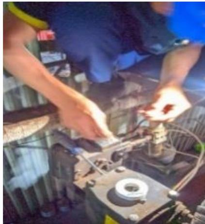
**Gambar 3.26 Perbaikan *Positioner Blowup Steam* Uap Boiler**
