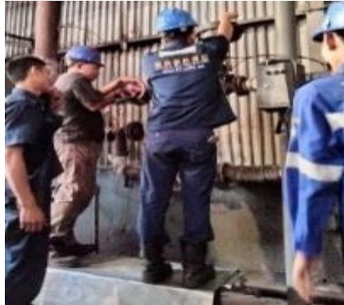
**Gambar 3.87 Perbaikan *Positioner Blowup Steam Uap Boiler***
