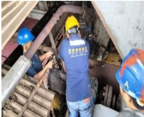
**Gambar 3.70 Pembongkaran Elektro Motor & *Gearbox Bunch Press Conveyor***
