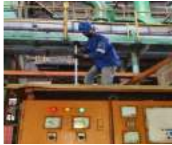
Gambar 3. 63 Cleaning panel station kernel & station press (Sumber : Dokumentasi 2025)
