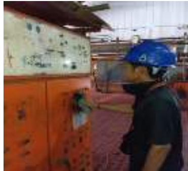
Gambar 3. 70 Cleaning panel station boiler (Sumber : Dokumentasi 2025)
