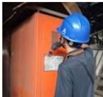
Gambar 3. 60 Cleaning panel station boiler (Sumber : Dokumentasi 2025)
