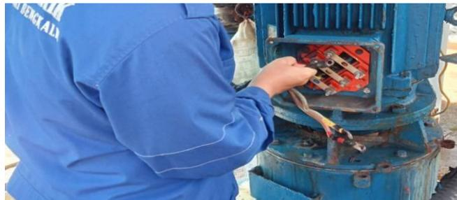
Gambar 3. 69 Connect power motor *grafiti tank* area WTP unit 2
