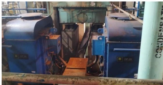
Gambar 3. 37 Preventif Maintenance motor 6KV di Cooling Tower.
