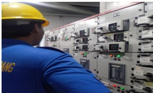
Gambar 3. 5 Inspeksi panel breaker area Coal Handling Control Building (CHCB)
