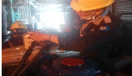
Gambar 3. 47 Preventive Maintenance motor MOV area turbin
