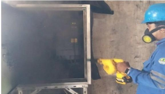
Gambar 3. 41 PM panel control di ruangan oprator CHCB
