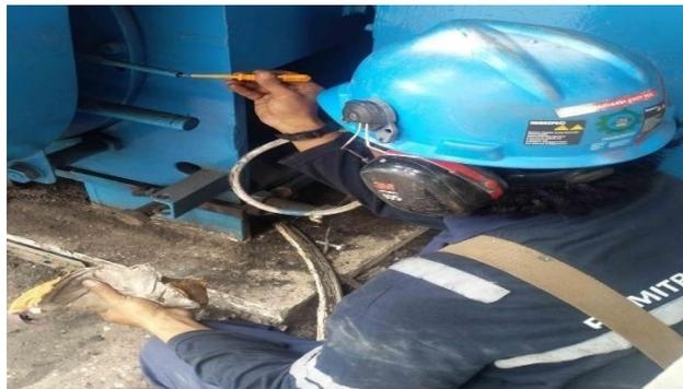
Gambar 3. 42 Greasing motor SAF, PAF, HPFF 1B, dan preventive maintenace di area Boiler
