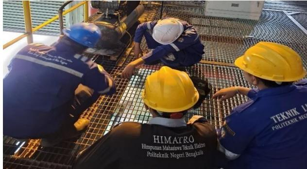
Gambar 3. 35 Pengetesan Compressor Busduct unit 2 dan top up oil compressor
