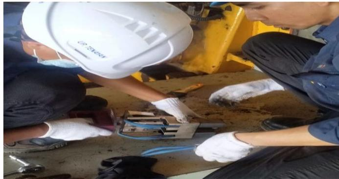
Gambar 3. 45 Pengecekan Hotspot carbon Brush Exciter generator unit.
