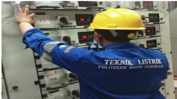
Gambar 3. 16 Pendataan Breaker Motor Control Center (MCC)
