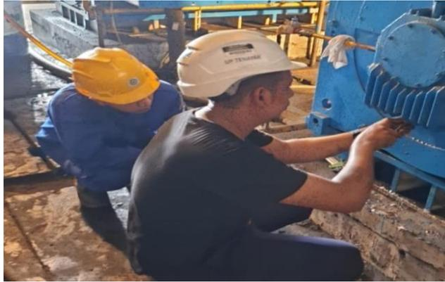
Gambar 3. 68 Progress Drain Oil motor BFP 1B, indikasi tercampur air
