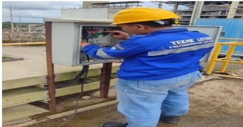
Gambar 3. 30 Support power 1 phasa untuk sipil di cooling tower area water treatman plant (WTP).
