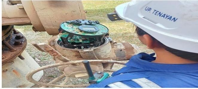
Gambar 3. 58 Pengecekan dan perbaikan motor operated valve (MOV)
