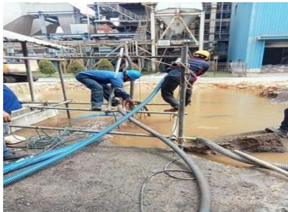
Gambar 3. 39 connect power sump pump 3 fase
