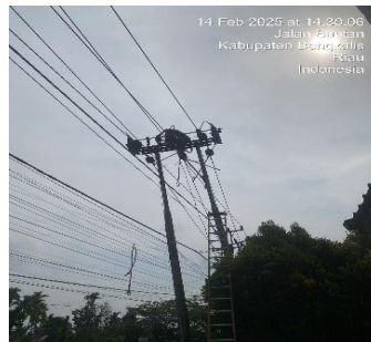
Gambar 3. 8 Pekerjaan pergantian Pin Insulator
