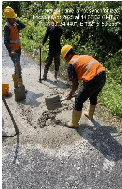
Gambar 2.84 Pengecoran manset
