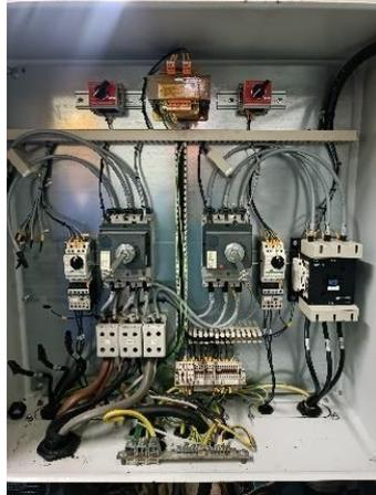
**Gambar 3.27** Panel Kontrol *Compressor Starting*
