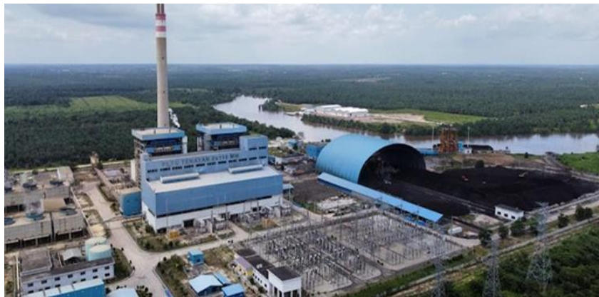
Gambar 2.1 Penampakan PLTU Tenayan (Sumber: https://www.ranahriau.com )
