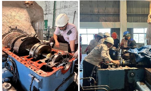
Gambar 3. 4 Overhaul Turbin 2 (Sumber Dokumentasi: PT. Power Plant)
