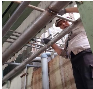
Gambar 3. 30 Repair line urea WWTP aerob (Sumber Dokumentasi: PT. Power Plant)
