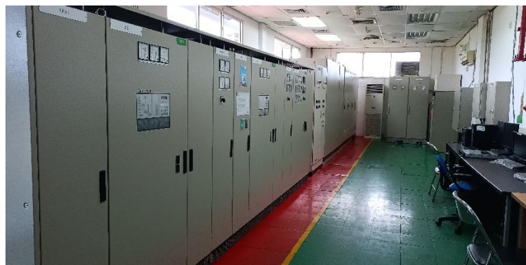
Gambar 4.1 Uninterruptible Power Supply (UPS) (Sumber: PT. Kilang Pertamina Internasional RU II Dumai)
