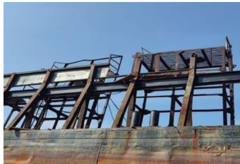
Gambar 2 31 Proses Repair Dinding Side Board
