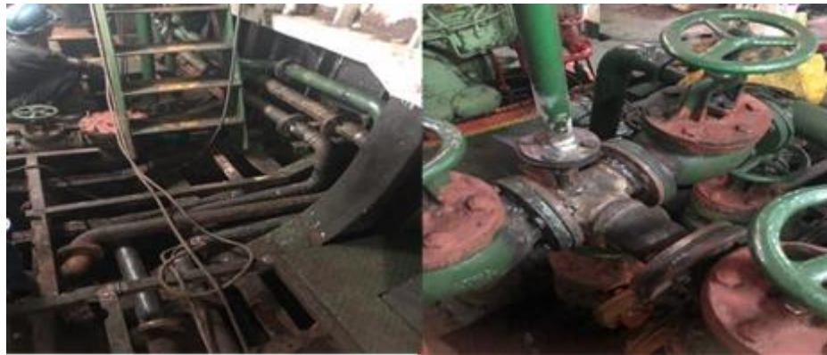
Gambar 2 57 Record Data Repair Pipa
