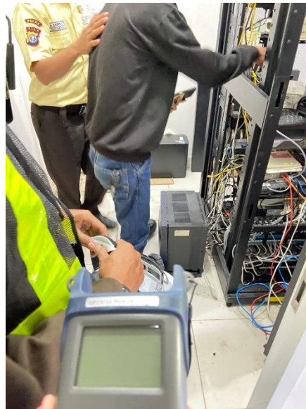
Gambar 3. 10 Pengecekan Redaman Di Splitter Toyota Astra Finance
