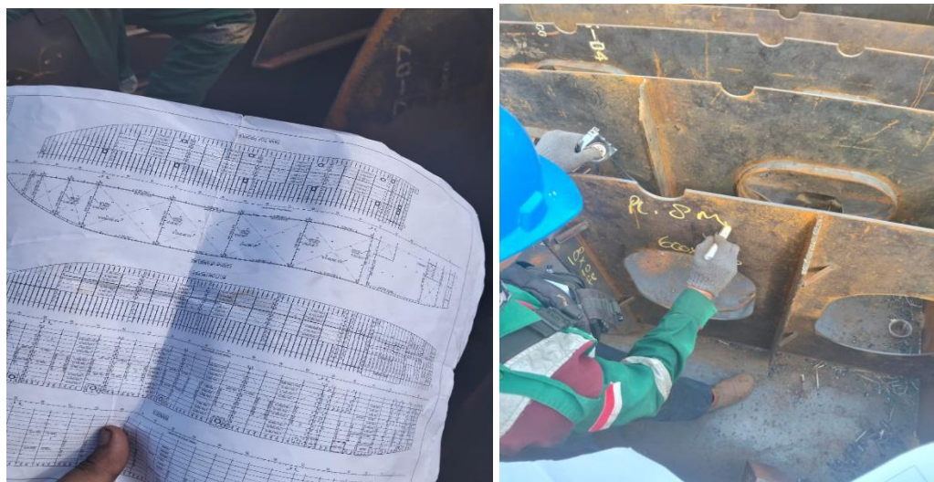
Gambar 3. 79 proses scantling KMP JAMBO frame -3 sampai 18
