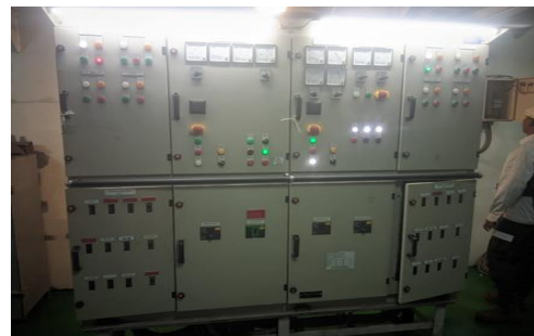
Gambar 3.7 generator diesel dan Main Switchboard
