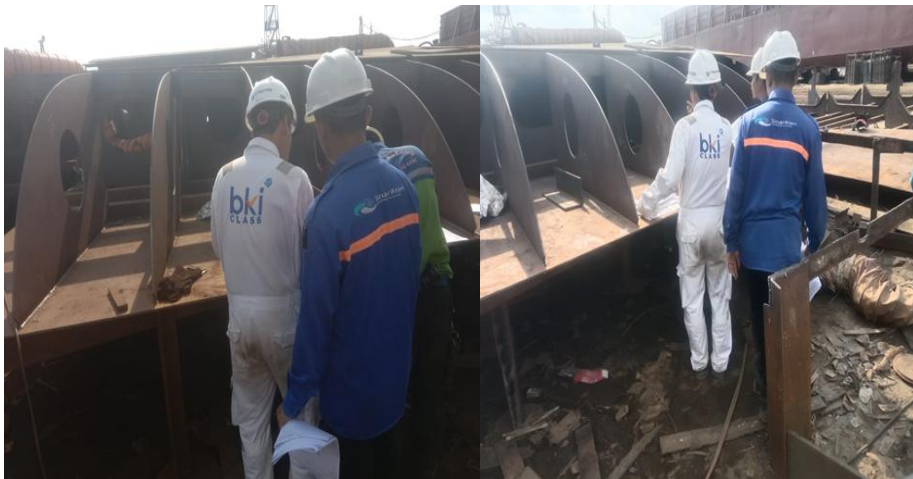
Gambar 3.1 scantling KMP JAMBO XV4
